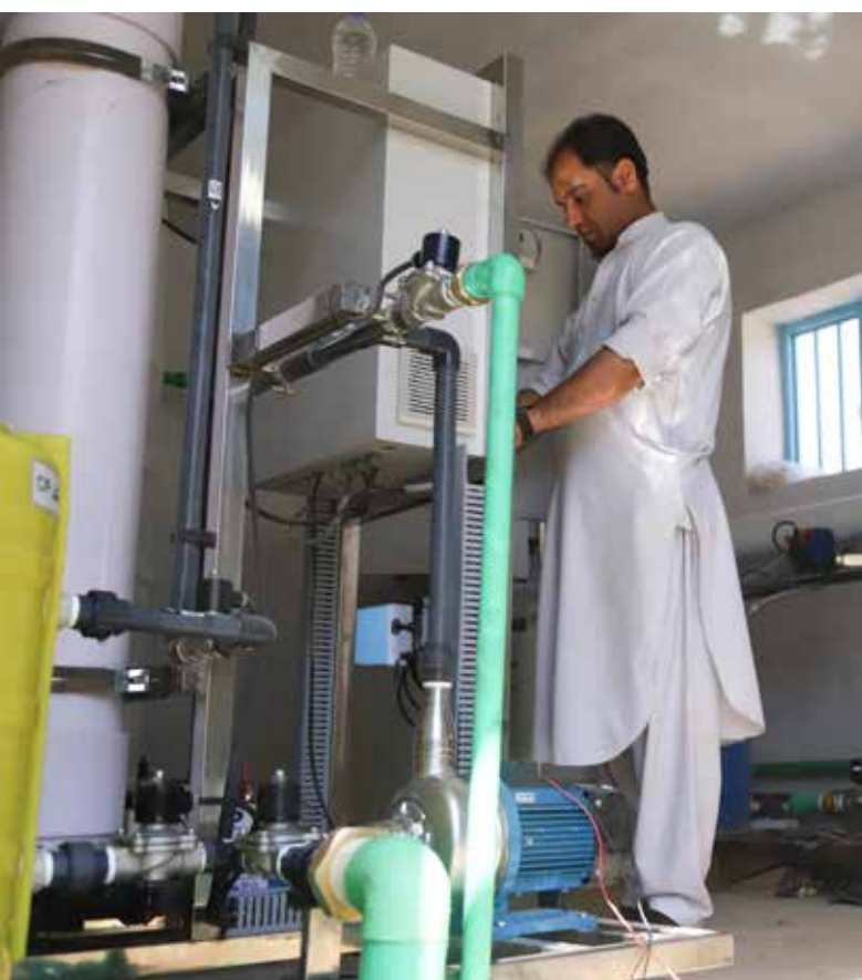
An innovative approach - an RO operator, unit and water treatment system - treating highly saline water to become a safe drinking source, powered by solar energy for sustainability. © World Vision Afghanistan
